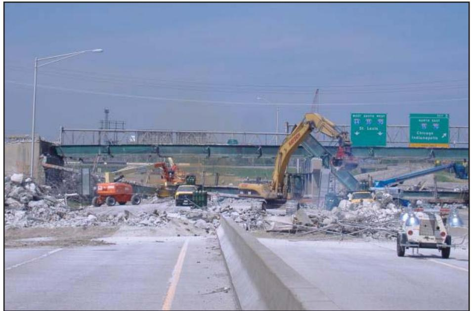
**Crews tear down the 9th and 10th street bridges over Interstate 64 in Illinois over a weekend. Over the next two years, Illinois DOT will be completing much of the work to tie in the tri-level with the new Relocated I-70. This will require regular lane closures, as well as some interstate and ramp closures.**
