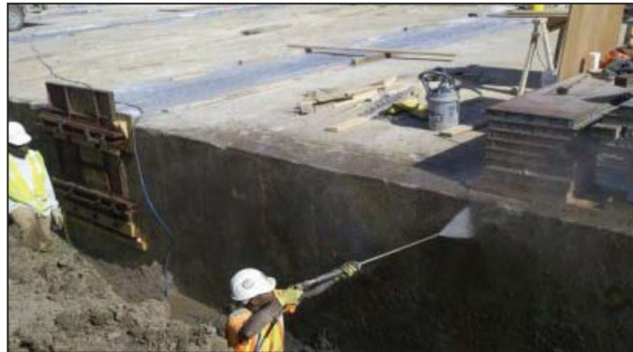
Laborers power wash concrete before constructing new formwork.
