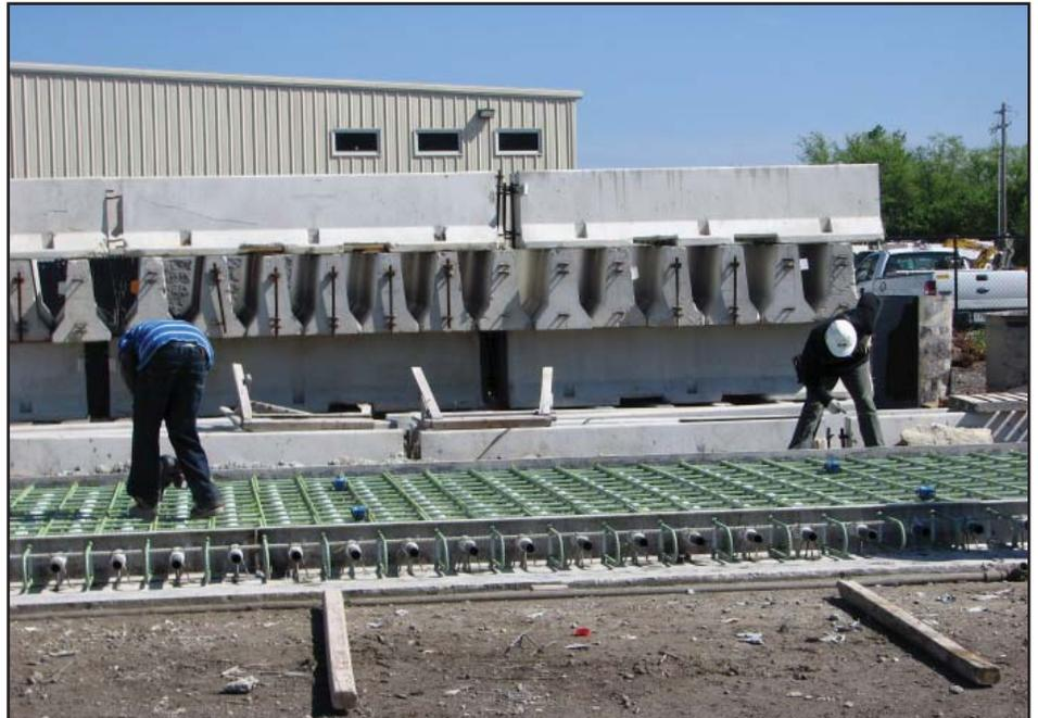
**XL Contracting workers tie together the reinforcing steel for a deck panel, a portion of the new bridge’s driving surface.**
