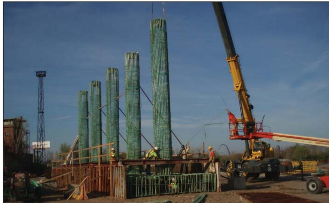
Crews set steel casings into position before placing concrete for foundation work for the bridge from I-64 to the relocated I-70.
