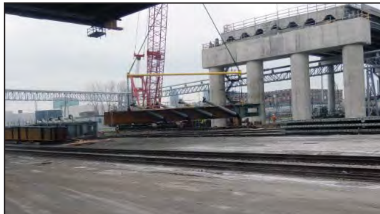
Lifting a girder off the ground ...
