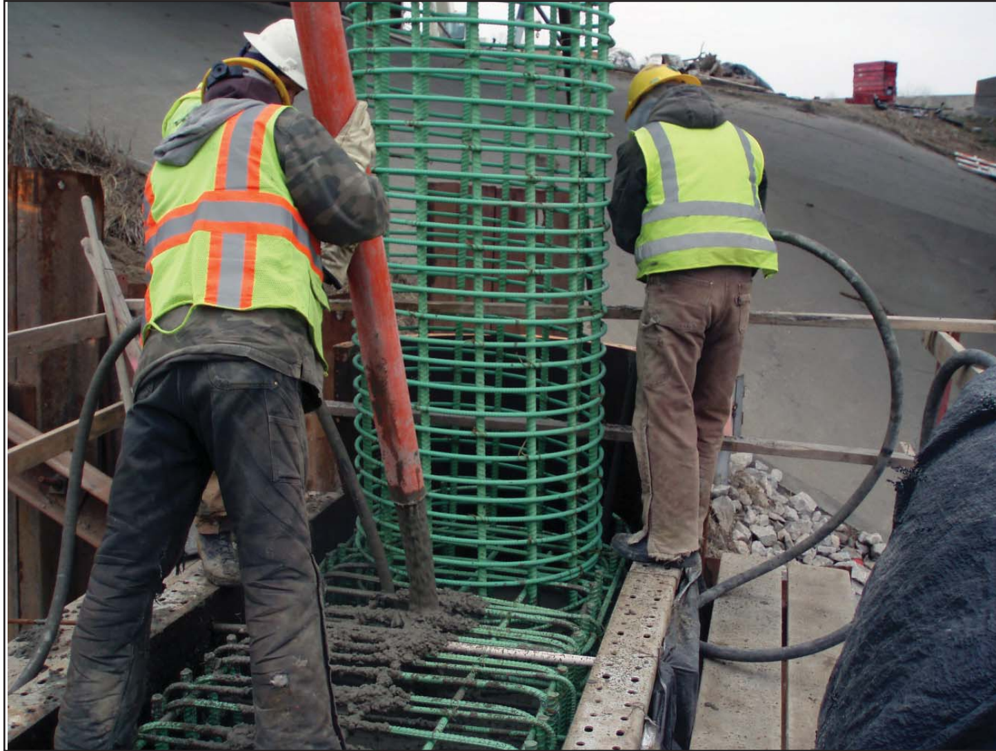
Workers place concrete for a bridge foundation in Illinois.
