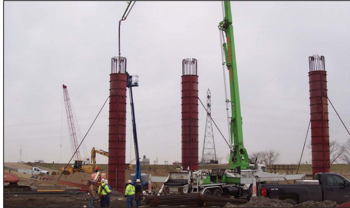
Construction on the Illinois Approach continues. Here, crews place concrete in the columns that make up a portion of the bridge foundation.
